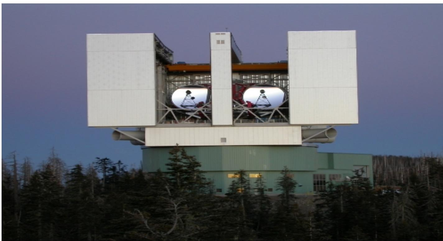
Large Binocular Telescope in Arizona (8.4m Mirrors, NIR-optical)
