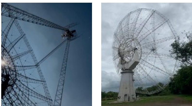
Fig2. Left: Antenna C3 of GMRT-NCRA, shows the dipoles and the receiver Right: Antenna C4 GMRT-NCRA, shows the entire structure. The base consists amplifiers and modulators.
