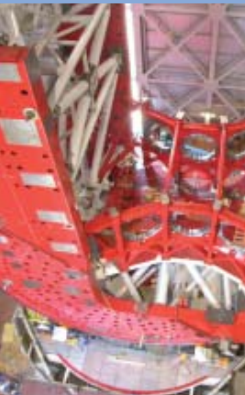
Above, the LBT superstructure, built in Italy and shipped to Arizona, is reassembled on Mount Graham.
